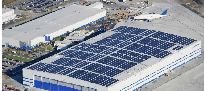
3 megawatt photovoltaic panels on 600,000 SF roof
